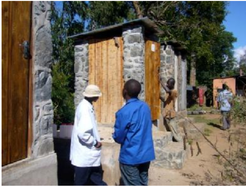
Testing effectiveness worm and terra preta toilet, June 2014
